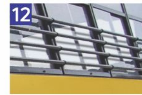
12 Window guard rails
