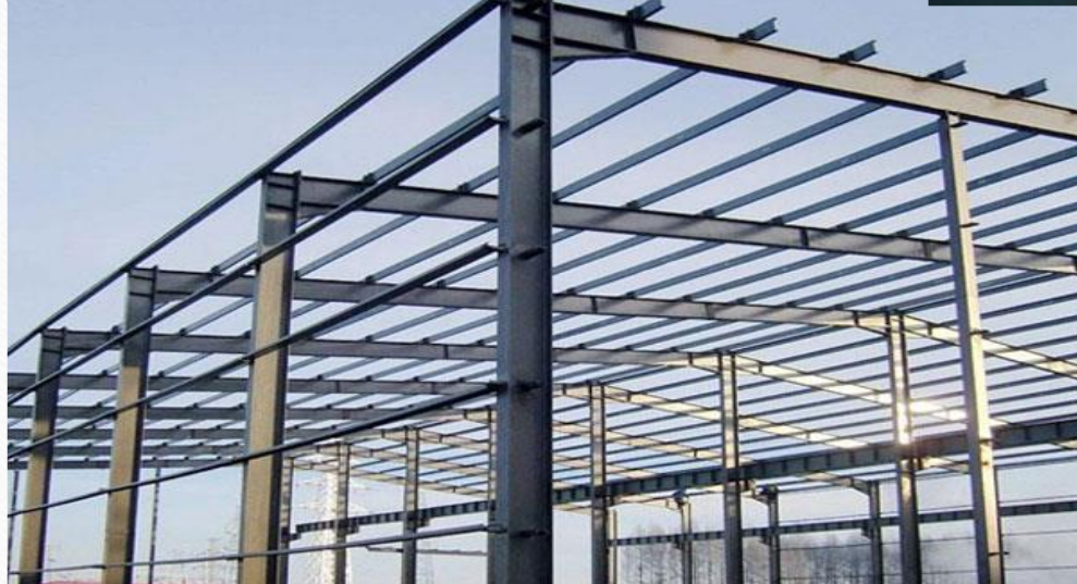
PEB Structure fabrication & Erection
