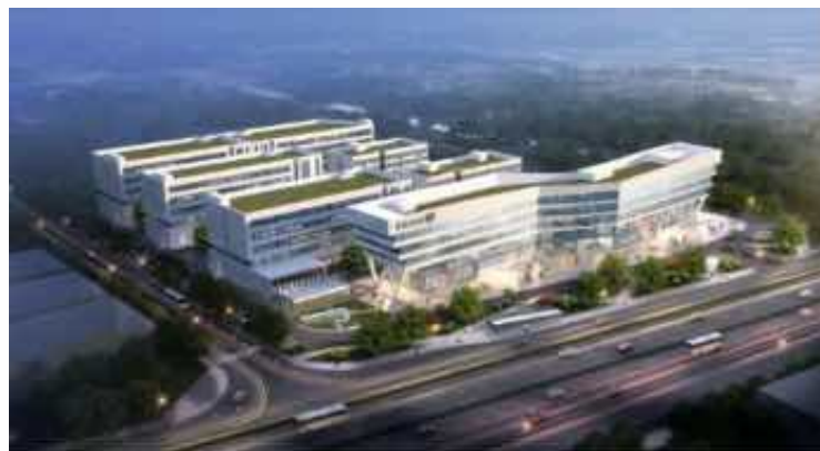
Changsha Manufacturing Base Plant
