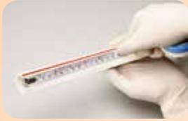
**MEASURING:** In order to make a proper and neat joint, we should measure the pipe length accurately and make a visible marking using a pen. Ensure that the Pipe and Fittings are compatible.
