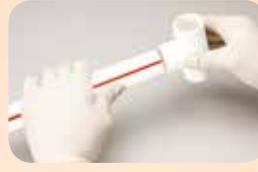
**FITTING PREPERATION:** Use a clean dry cloth, wipe the dirt and moisture from the Fittings, sockets and Pipe. Dry fit the Pipe to ensure total entry into the bottom of the Fittings socket and make a visible marking using a dark pen.
