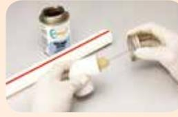
**SOLVENT CEMENT APPLICATION:** Use only APL Apollo CPVC Cement to ensure a perfect solvent weld joint. When making a joint, apply an even coat of cement on the Pipe end & also inside the Fitting socket.
