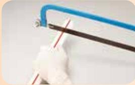
**CUTTING:** We can cut the Pipe easily with a sharp saw/cutter. Cutting the Pipe as squarely as possible (at 90°) provides optimal bonding area within a joint.
