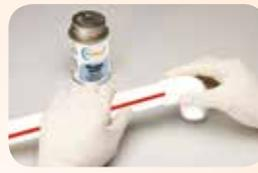
**ASSEMBLY:** Immediately after applying the solvent, insert the Pipe into the socket. Rotate the Pipe ½ or ¼ while inserting. This motion ensures an even distribution of cement within the joint. Properly align the Fittings and leave it for
