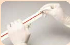
**DEBURRING/BEVELING:** Burrs in and on end can obstruct flow or proper contact between the Pipe and socket of the Fitting during assembly and should be remove from both in and outside of the Pipe.
